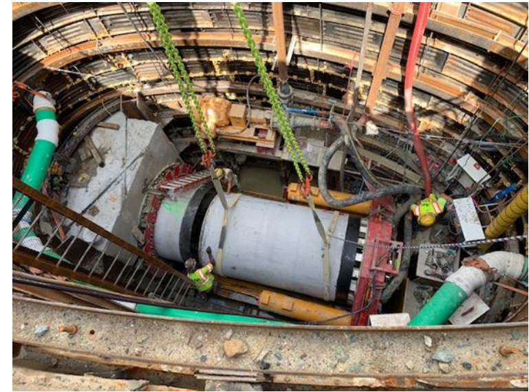
Micro Tunneling Machine Setup
