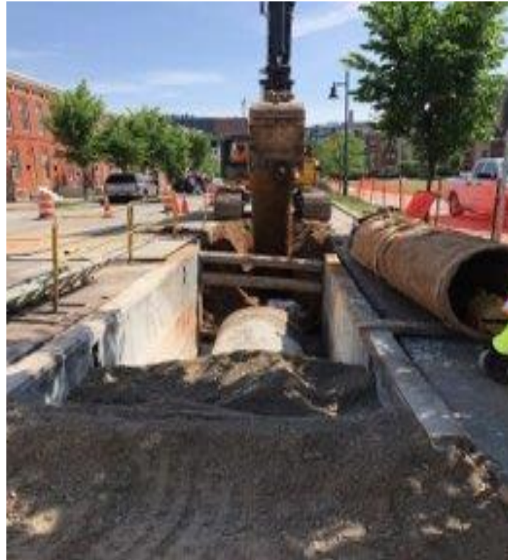
Removal of Existing Sewer Pipe
