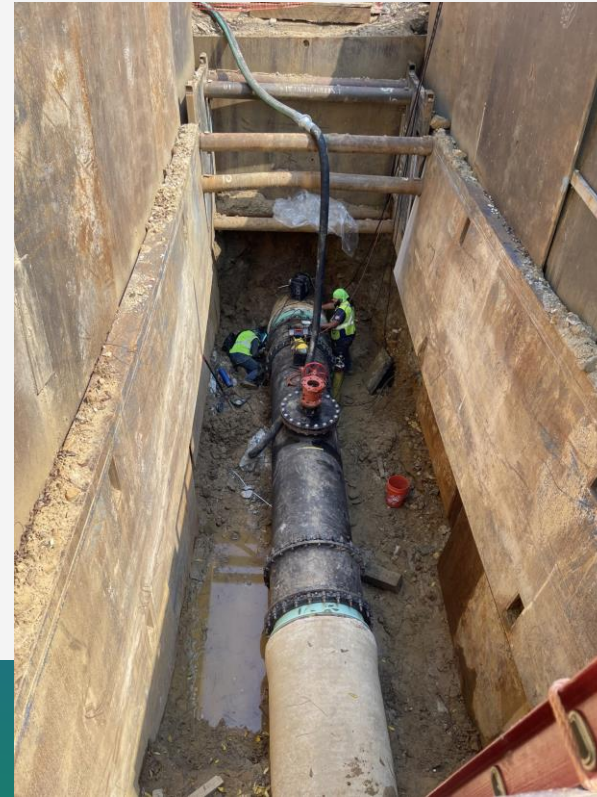
36" PCCP Damaged Pipe Replaced with DIP w/ Access
