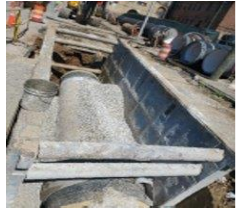
Pressure Sewer Pipe Installation
